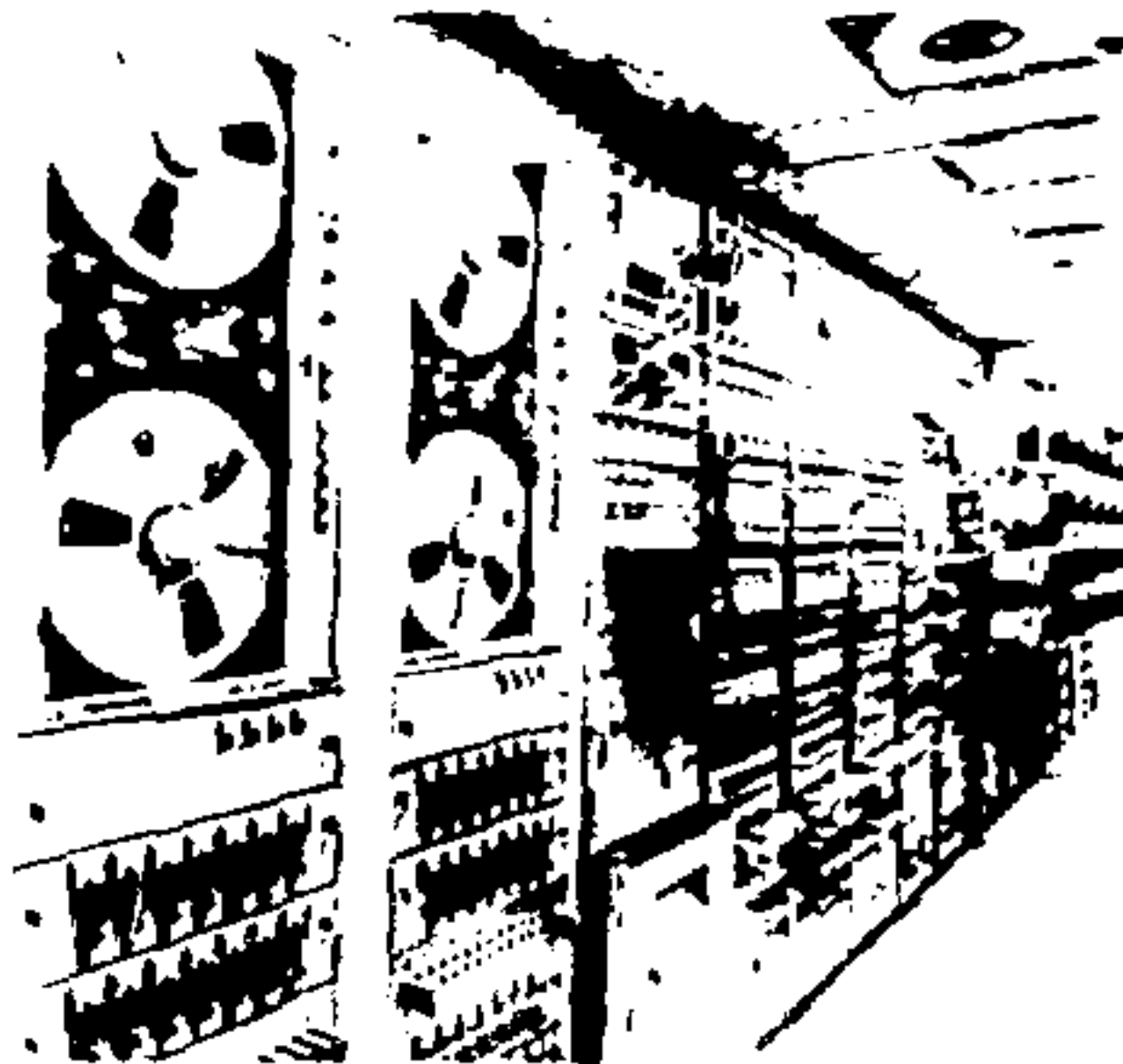
Figure 1. Typical multichannel instrumentation in mobile station for recording of underground test data
