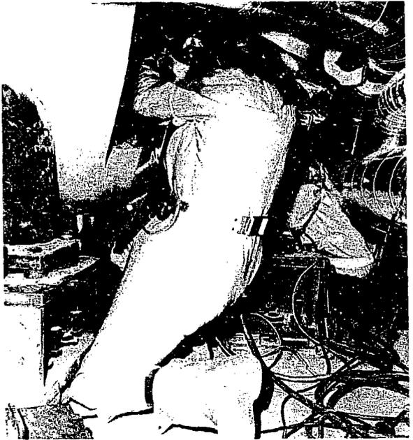
in the various repair aspects of leaking tube identification, inspection, plugging and testing within the radioactive and confined environment of a boiler head (see Figure 3) was immediately available. Within five days the unit was back on line; the leak (a hole approximately .254 mm in diameter) had been found within the 2600 tubes totalling 1858 m<sup>2</sup> of surface, plugged and tested.
