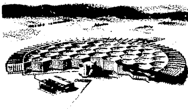
Fig. 12. A mirror fusion reactor with a fan-shaped expander and periodic focusing direct converter.
