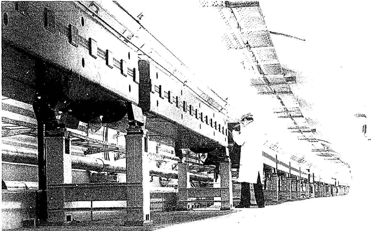
*An arc of the SPS ring showing bending magnets and focusing quadrupoles in place. (CERN 10.11.74)*
