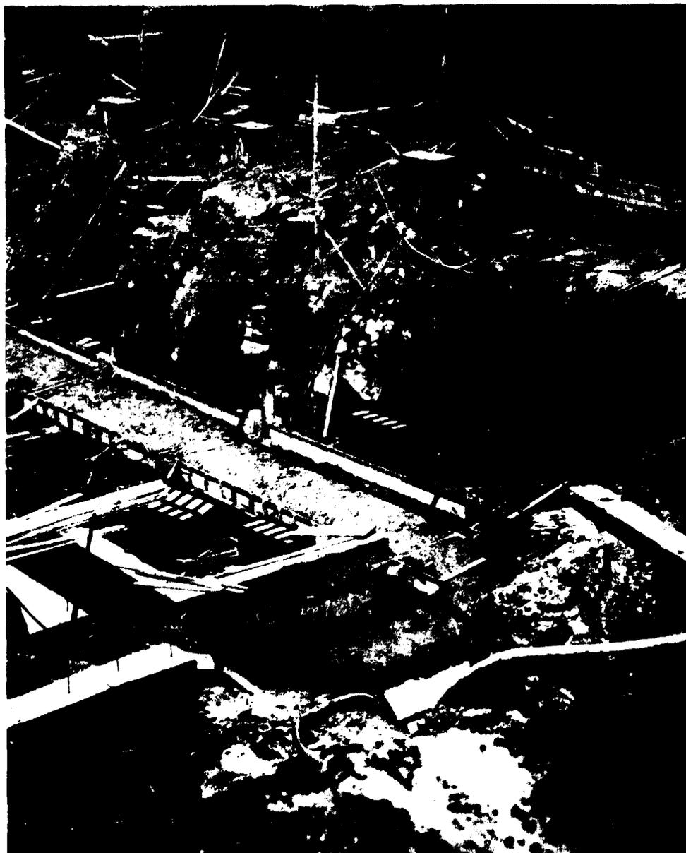
Fig. 18a. Apparently stable rock slope a couple of months after blasting and excavation. Several weeks afterwards, when the building was partly finished, steep zones of clay-weathered rock moved out in a semi-liquid condition (196).
