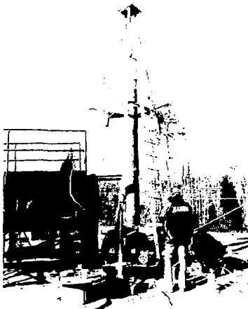
Fig. 18. Heater Suspended on A-Frame Preparatory to Insertion
