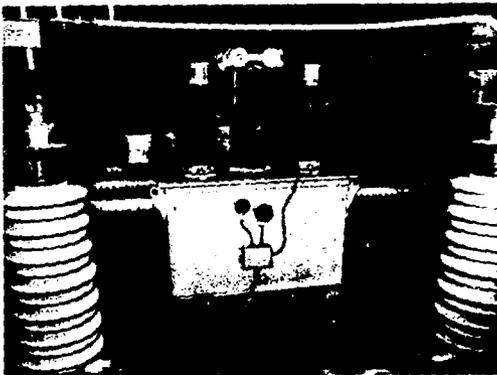
Fig. 3. Power-isolation transformer
