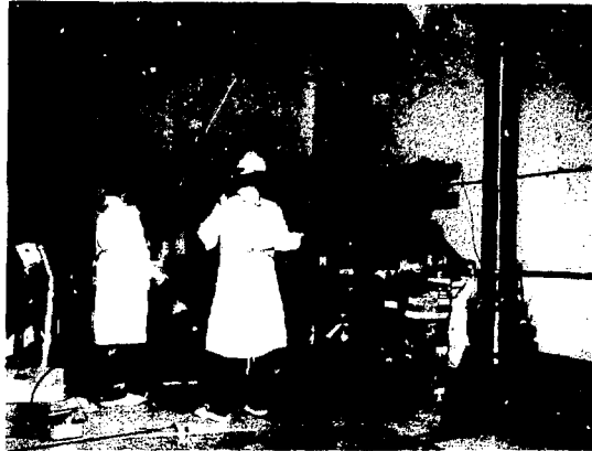
Fig. 9. Remote cutting of unnecessary supports to minimize waste container size.
