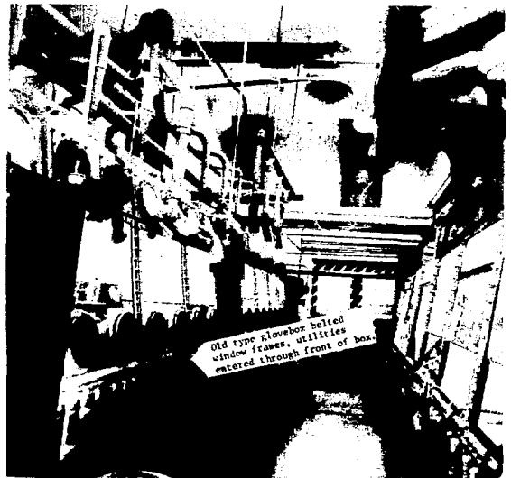
Fig. 31. Gloveboxes in room 308.
