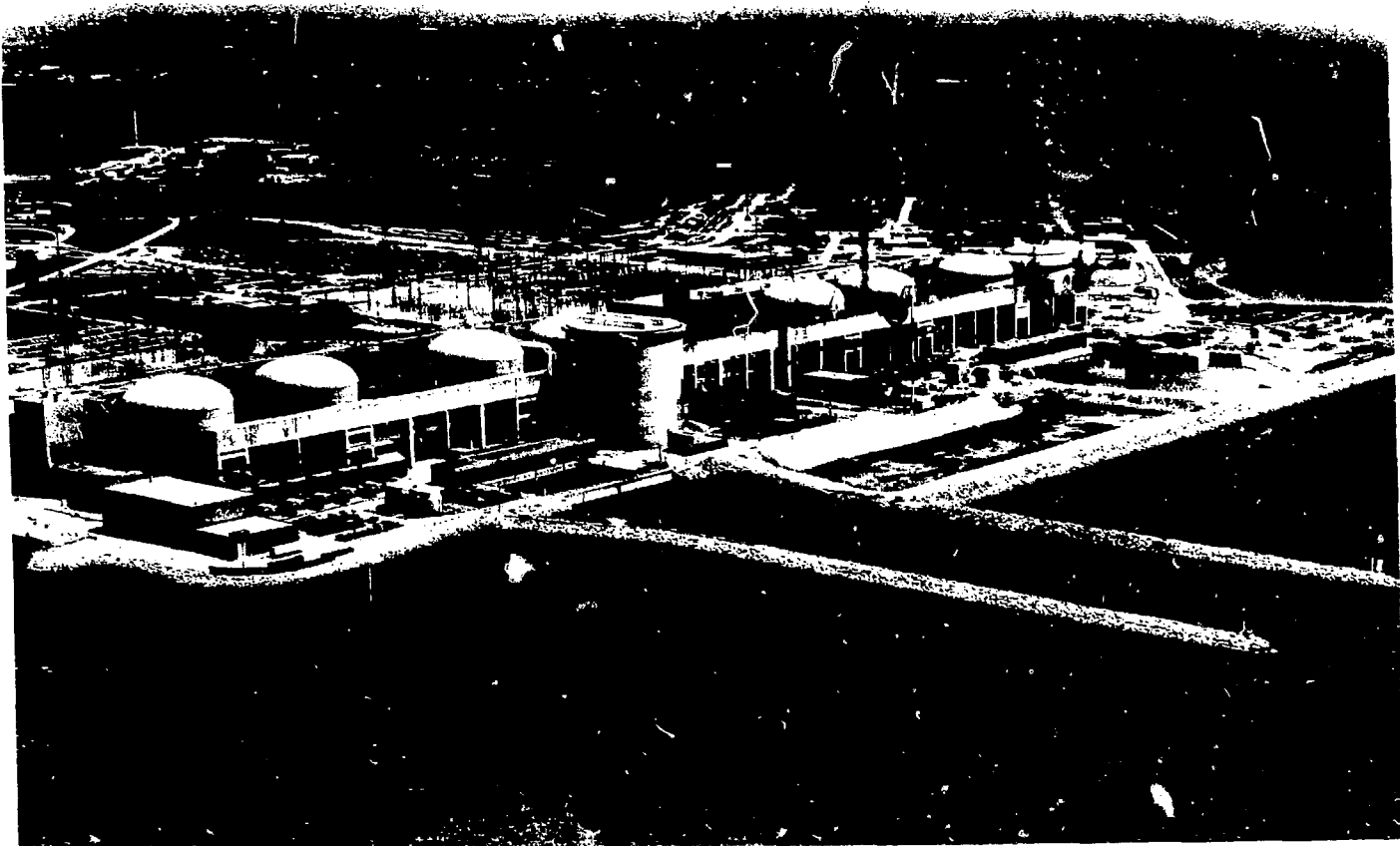
FIG. 2 VIEW OF THE PICKERING NUCLEAR GENERATING STATION IN MAY 1981.
