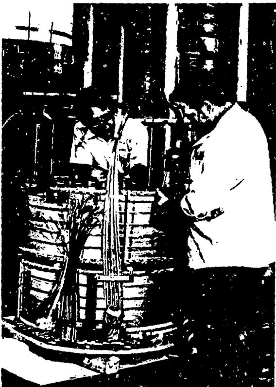
Fig. 2. A 3 MJ, 10 kA superconducting pulsed coil
