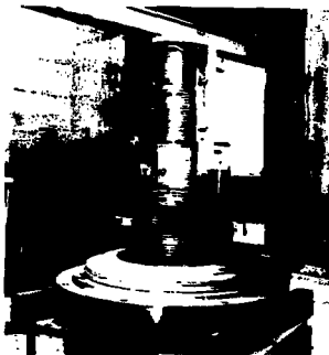
Fig. 5 Solenoid being assembled
