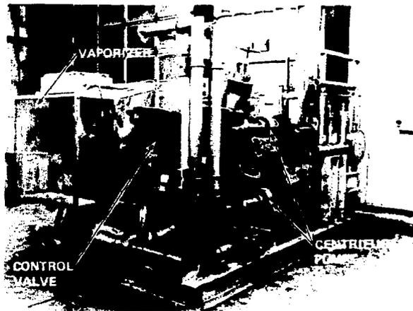
Fig. 3. Pump station (photo courtesy of Cryogenic Engineering Company).
