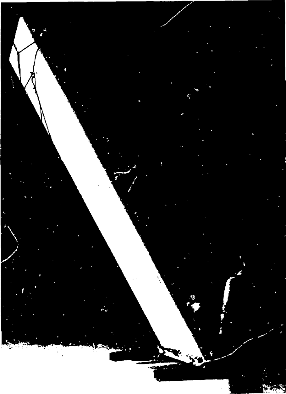
Fig. 5. Winching the support to a vertical position.
