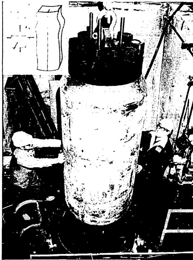
Fig. 2. Test vessel used for preliminary thermal hydraulic tests (PTSE-0) being lowered into shroud.
