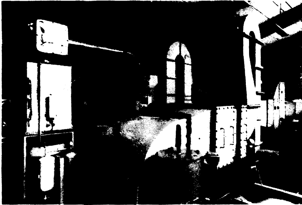
Figure 4. Filter installation at DR 3. In the foreground HEPA-filter F2 is seen; in the left-hand background HEPA/charcoal-filters F7/F9 are seen (cf. figure 3).
