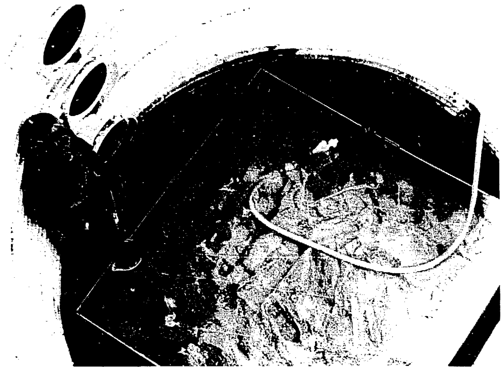
Fig. 14. Emplacing a metal frame in Caisson E to be used to position the Ottawa sand layer (frame was removed after the sand was added and compacted).
