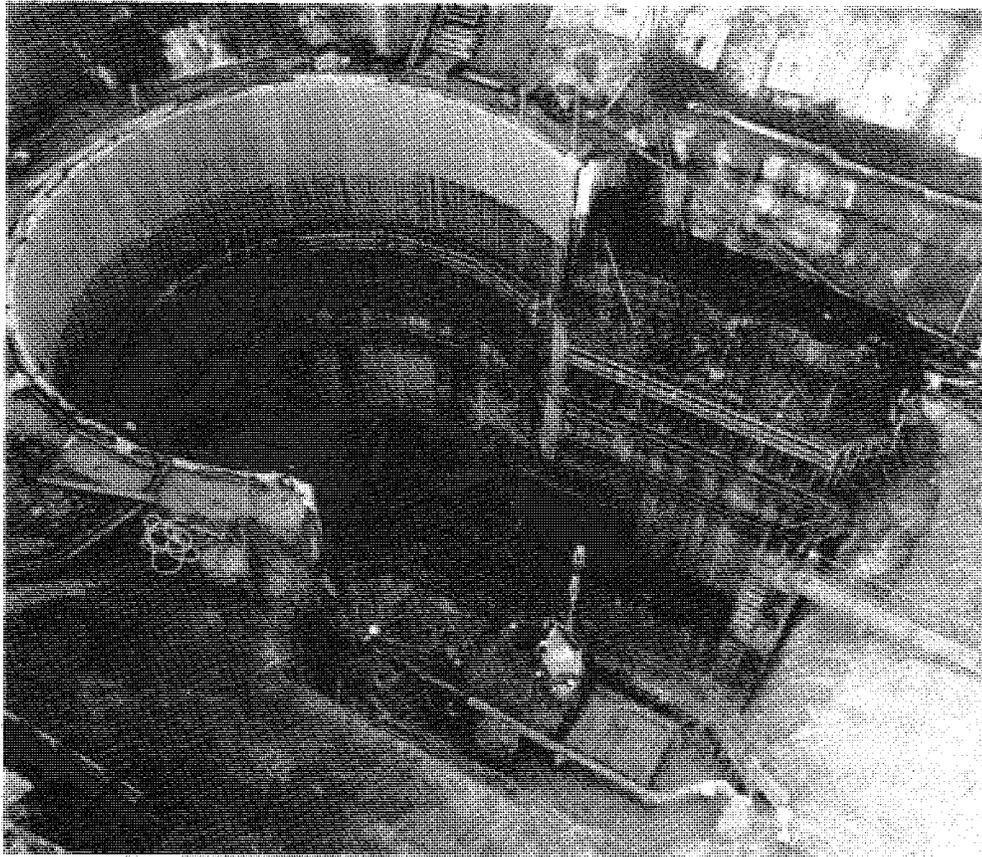
**Plate 2** Part of the open excavation for the UA1 detector hall. The photograph shows the 'garage' area where the detector was assembled. The SPS tunnel covered with earth crosses the bottom right-hand corner. During the 1980 shutdown the tunnel wall was opened and the second half of the detector hall was excavated.
