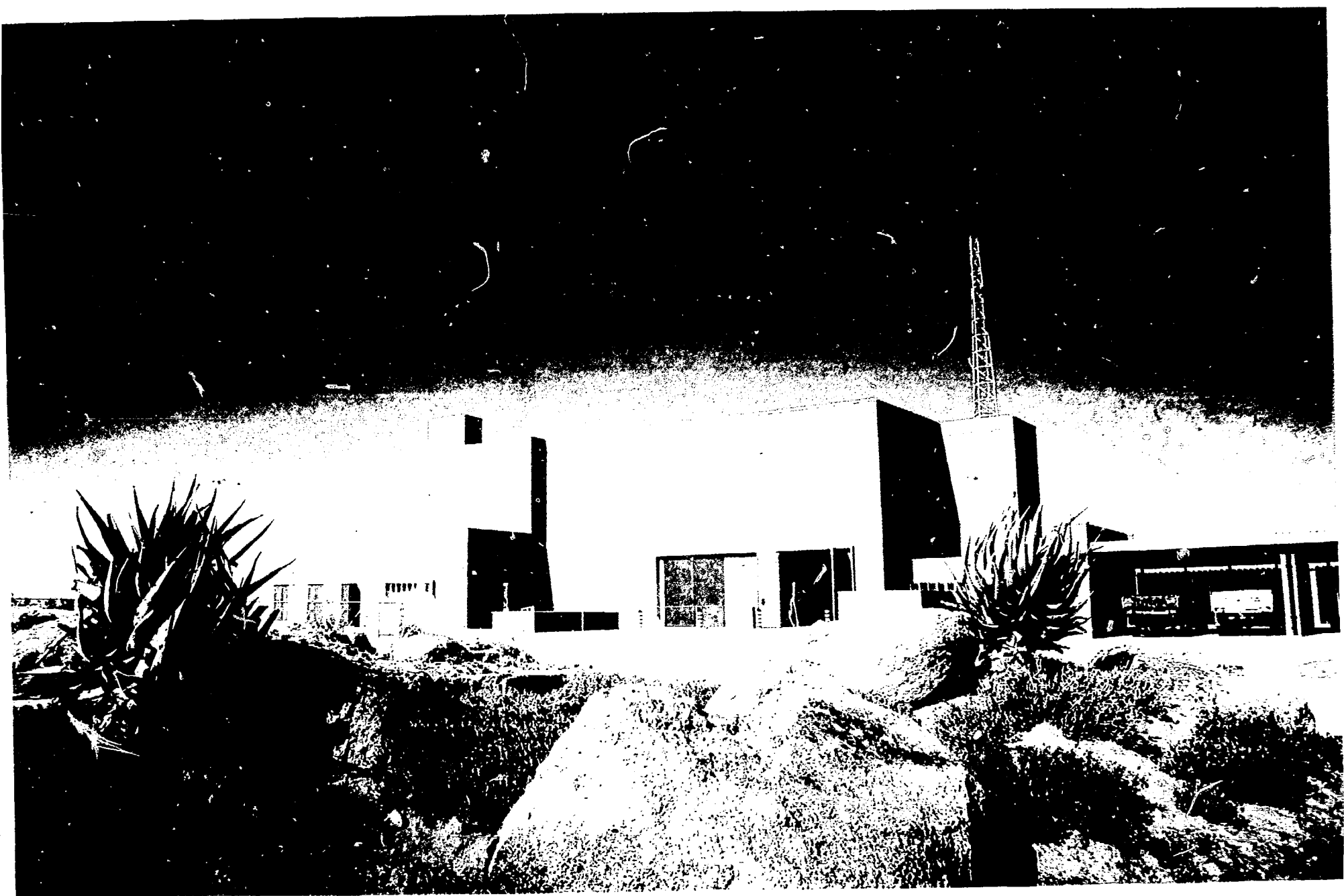
Waste disposal facility building at Vaalputs
