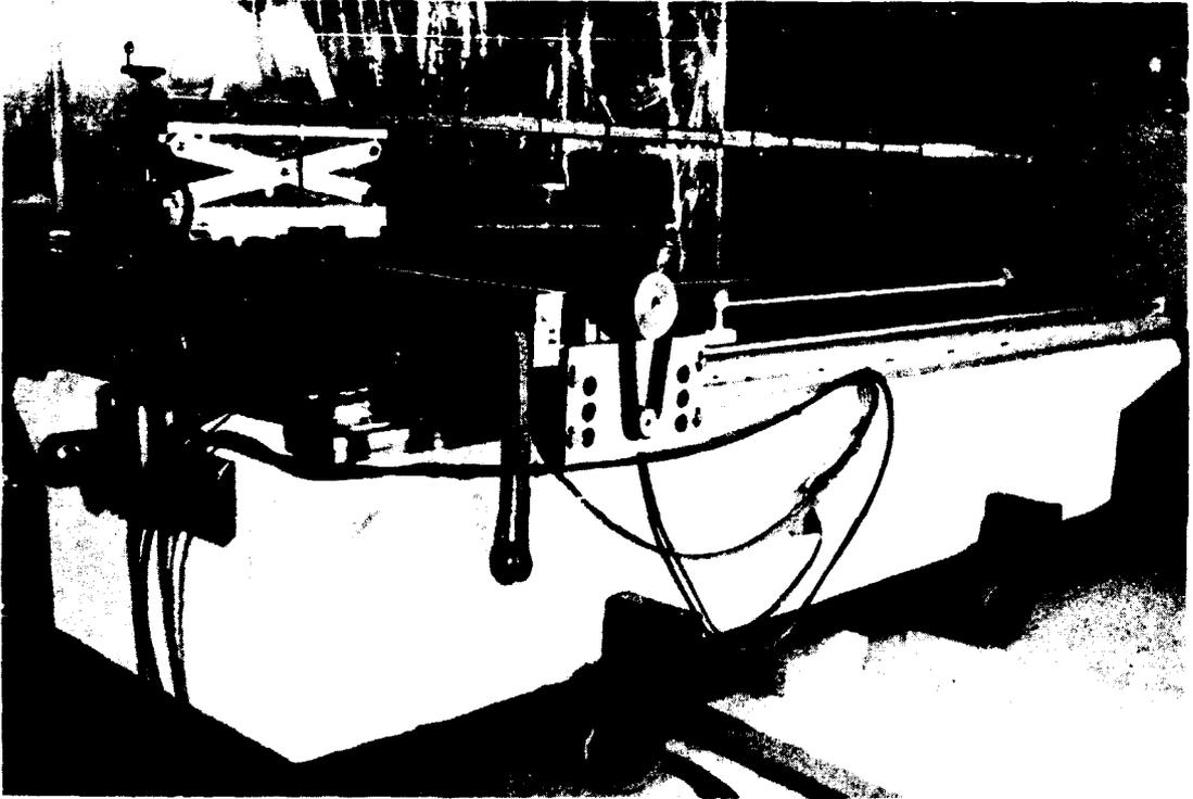
Fig. 3 The magnetic field measuring table for mapping the spectrometer. 16 Hall probes are carried on the T-shaped end of the measuring arm.
