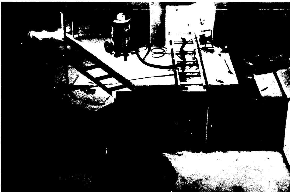
Fig. 1 View of the collimator tunnels at the north end of the experimental hall, showing the rails on which the steel collimators will travel.
