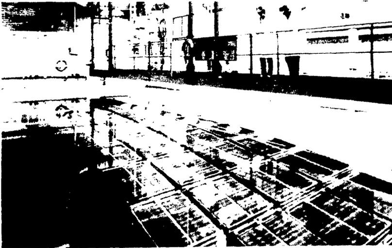
Bundles of used fuel in a water-filled storage pool at Ontario Hydro's Bruce Nuclear Power Station
