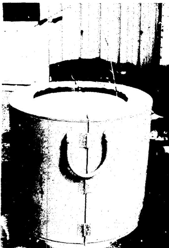
**Figure 5.3** A clam-shell type drum heater used to initiate the polymerization of a treated 55-gallon drum of compacted waste.
