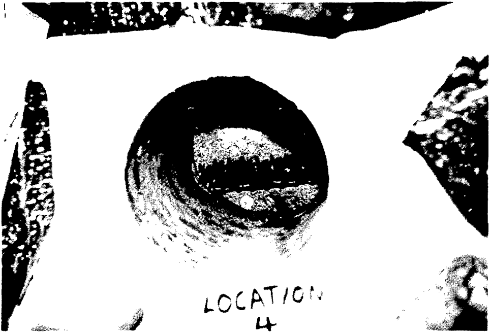
Fig. 6 Intersection of core drill with a reinforcing bar at site 4
