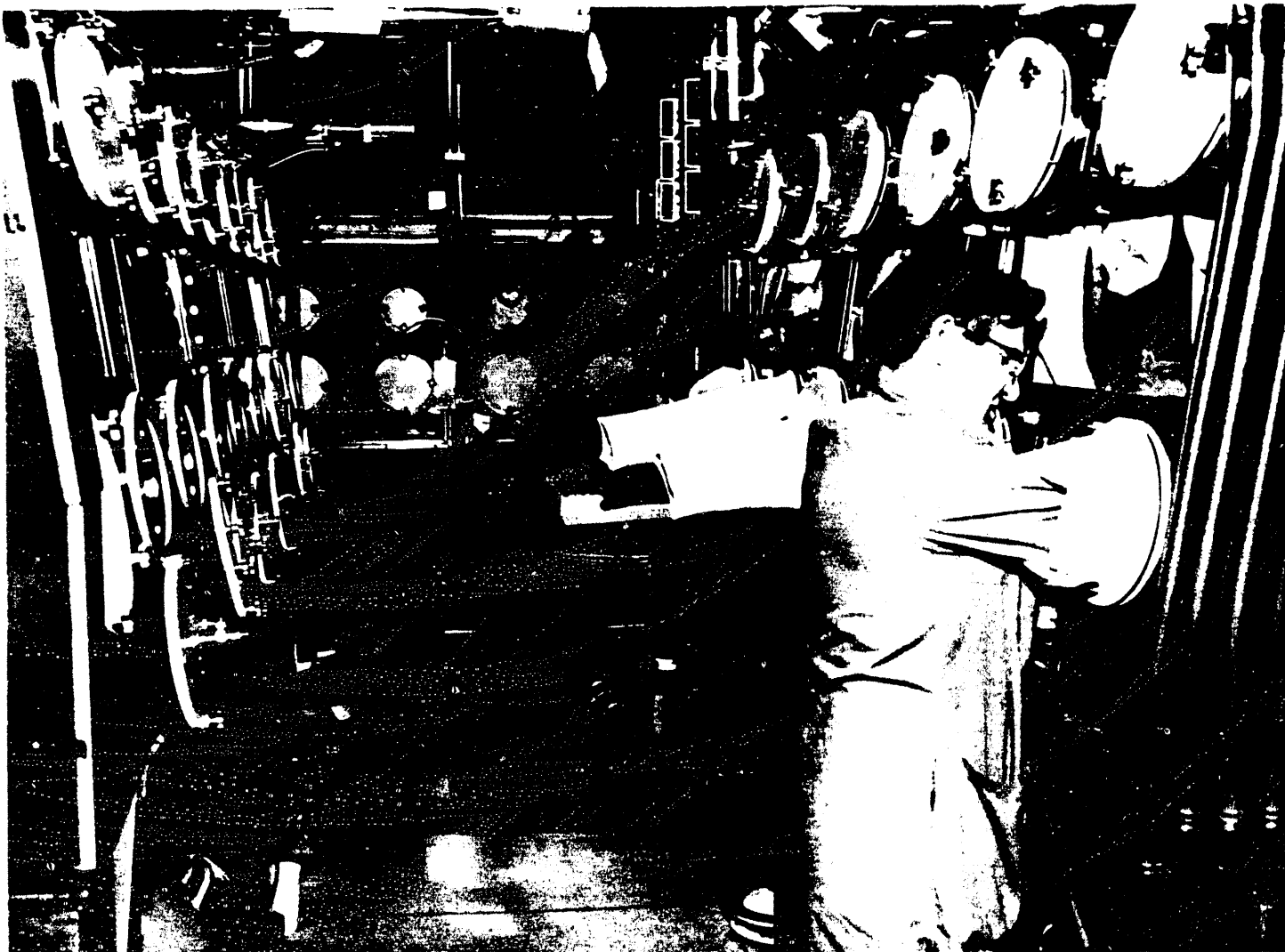
Fig. 2. An operator in LLNL's Material Processing Laboratory manipulating a stationary furnace component through gloves.
