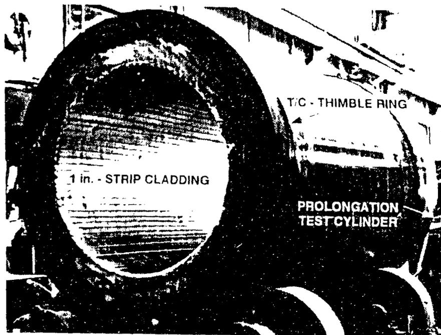
Fig. 6. Test-cylinder/prolongation assembly showing strip cladding before machining.
