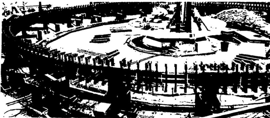
Fig. 2 The 15.1 meter diameter g-2 outer solenoid at the completion of winding
