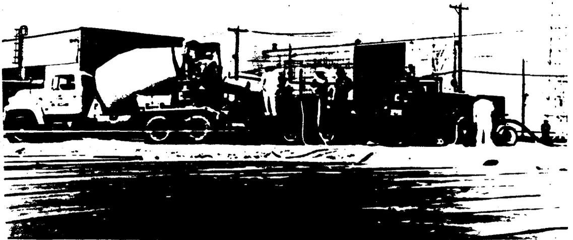
FIG. 4--The grout delivery system used during the field demonstration in May 1992.
