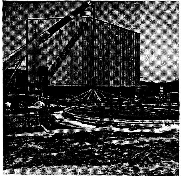
Fig. 3 Outer Coil is Removed From Building
