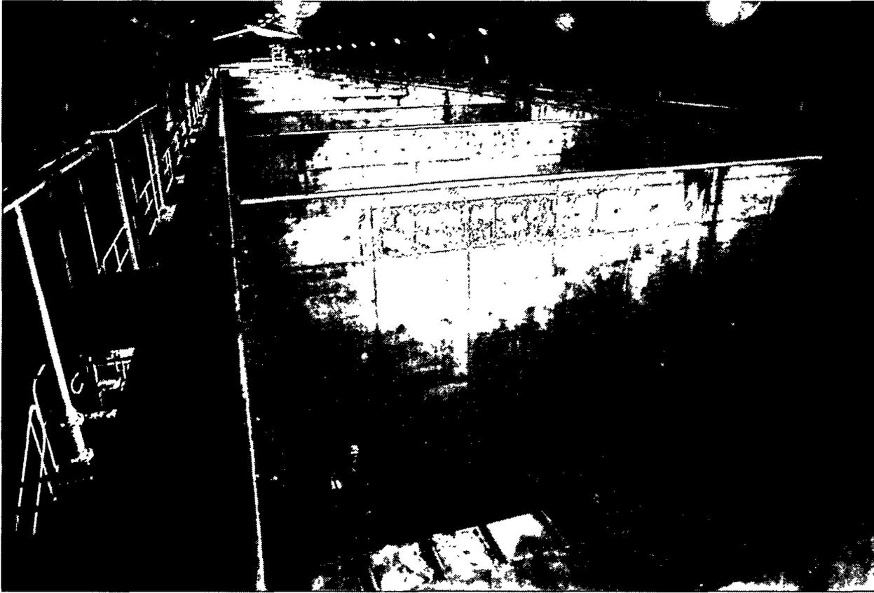
**Figure 10.** SFR divides its vaults into pits that contain the grouted waste packages (courtesy of SKB).
