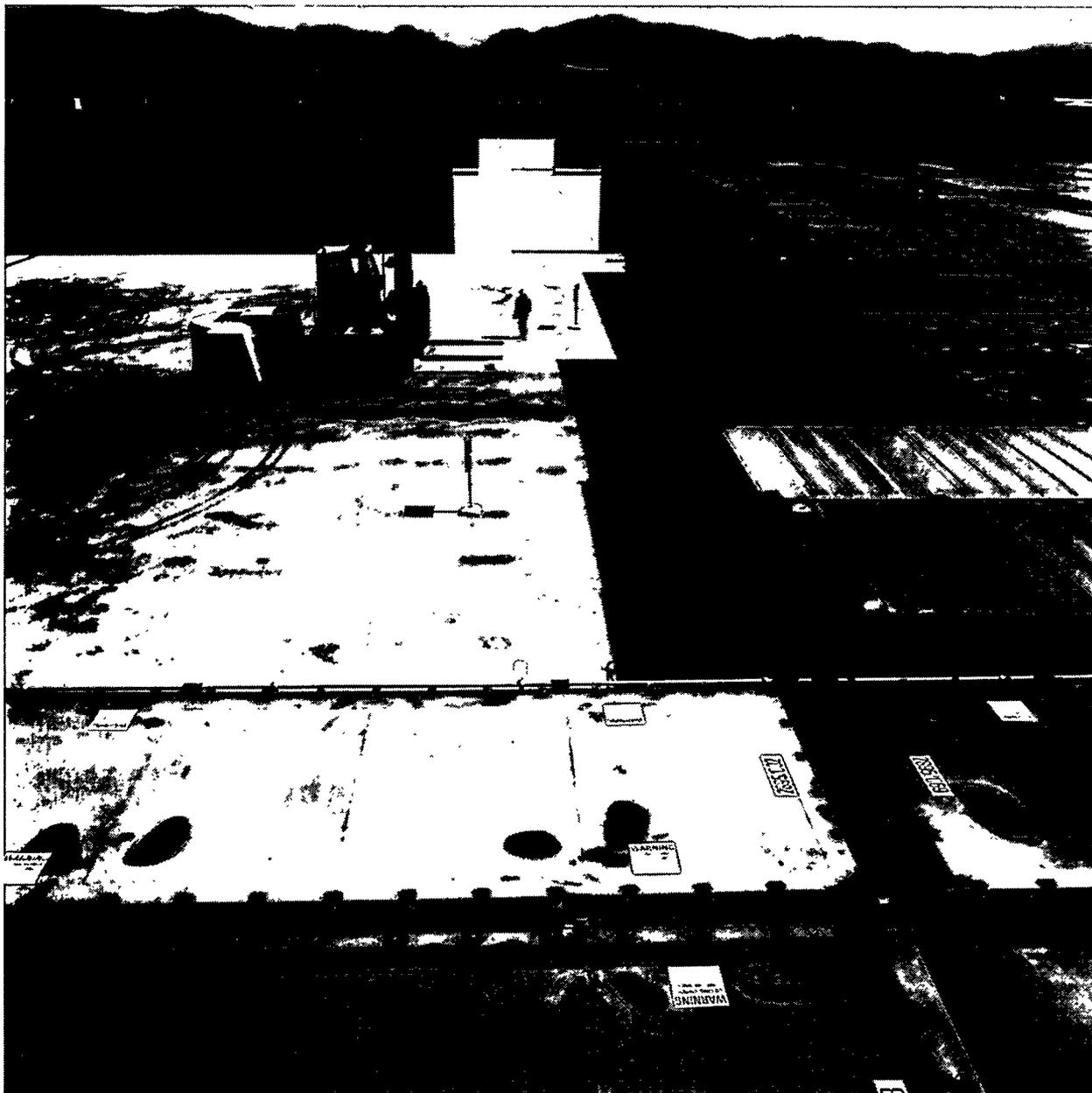
**Figure 12.** Engineered concrete vault at BNFL's LLW disposal site at Drigg (courtesy of BNFL).
