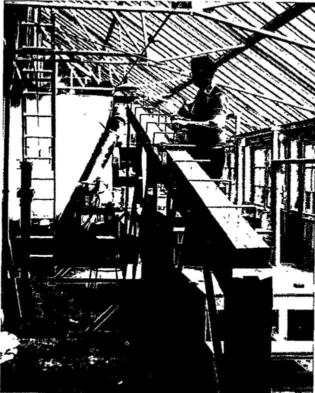
Fig. 23. Large soil beam used for final selection of diatomaceous earth as conductive-layer material. Lead bricks were placed on top of diatomaceous earth to simulate overburden.
