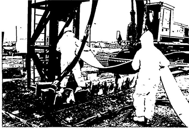
Figure 6. Lasagna® demonstration project installation.
