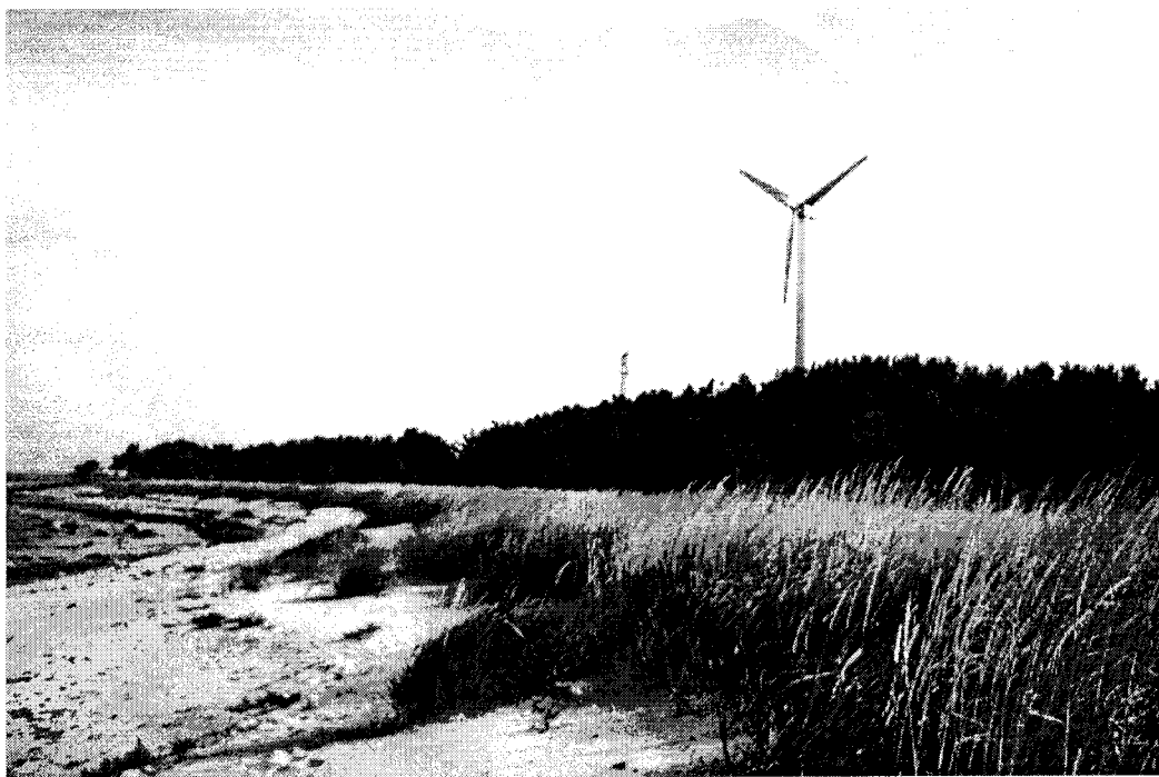
Fig. 3. The first wind turbine GENVIND CV – 150 kW in Estonia, Hiiumaa, Cape Tahkuna.
