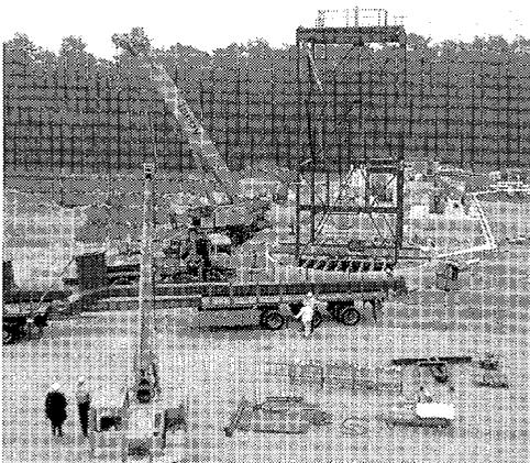
**Figure 10** Construction of the hoisting equipment for shaft sinking.
