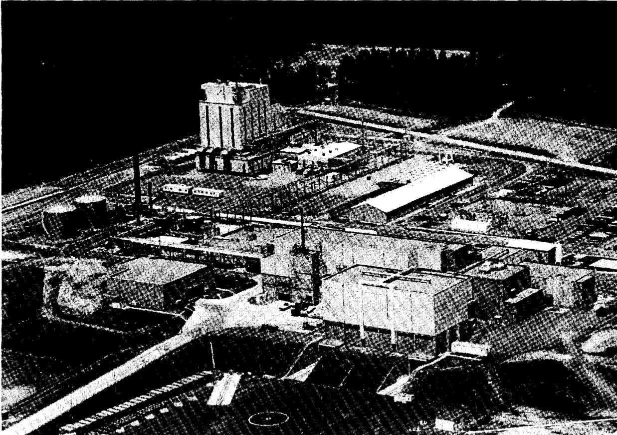
*Figure 1. The Barnwell Nuclear Fuel Plant. The cluster of buildings in the right foreground — the Separations Facility, the Fuel Receiving and Storage Facility, the Plutonium Nitrate Loading Station, and the Hot and Cold Laboratory Area — formed the heart of the plant.*
