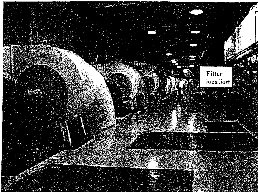
Possible location for installation of FVS (B-304)
