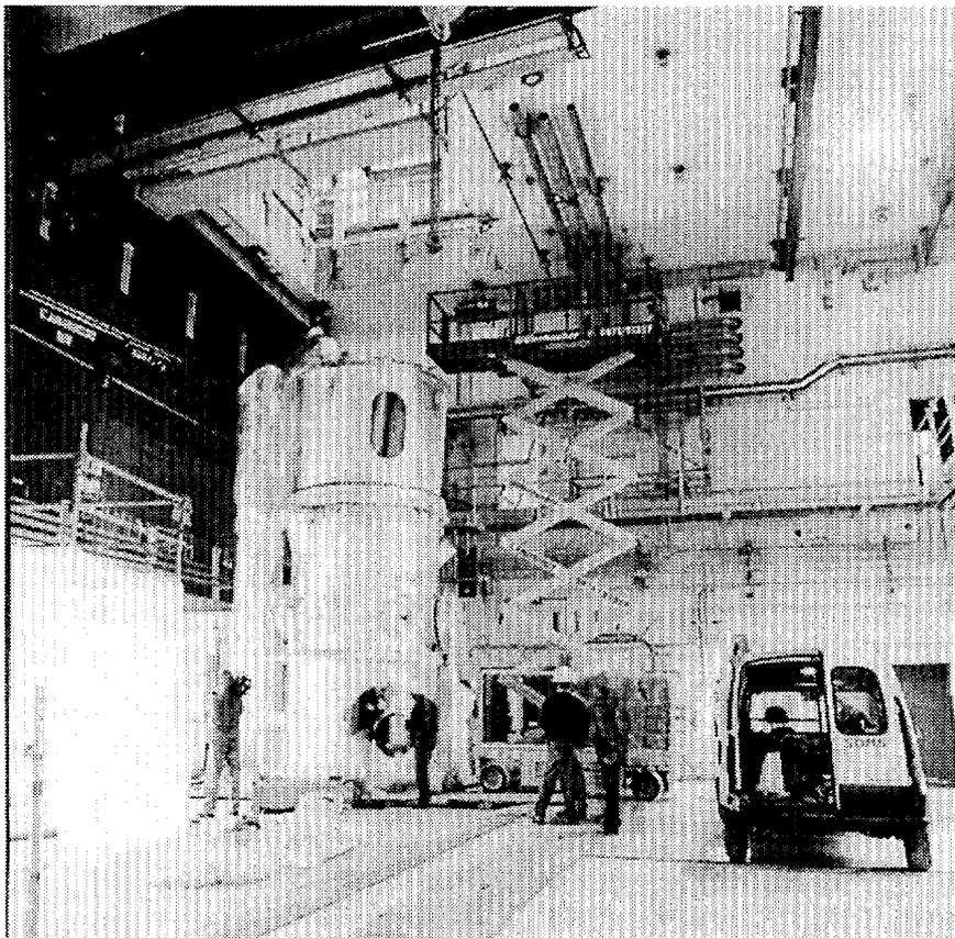
Figure 4: Moderator tank as arrived in the experimental hall of the FRM-II, ready for installation in the reactor pool.
