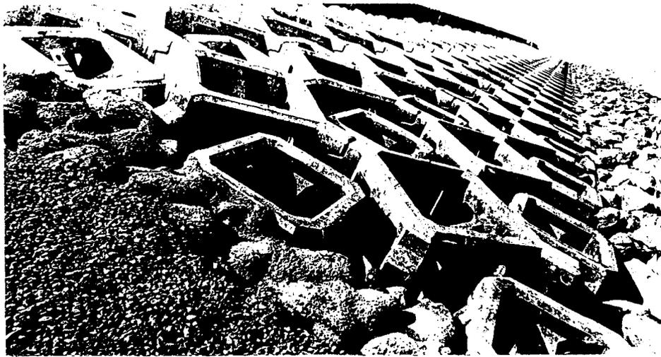
FIGURE 7: Diode Units
