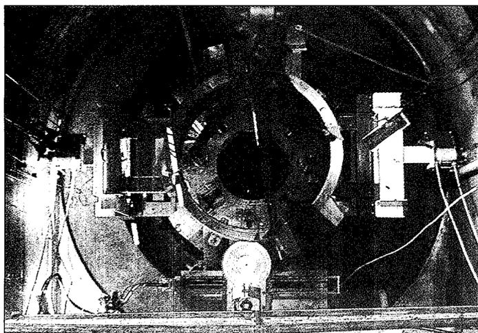
*Reactor pressure vessel horizontal cutting with anti-vibrations systems.*
