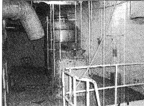
*Dismantling of valves and pipes of the pressuriser and of the Spray Tank.*
