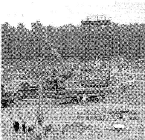
**Figure 10** Construction of the hoisting equipment for shaft sinking.
