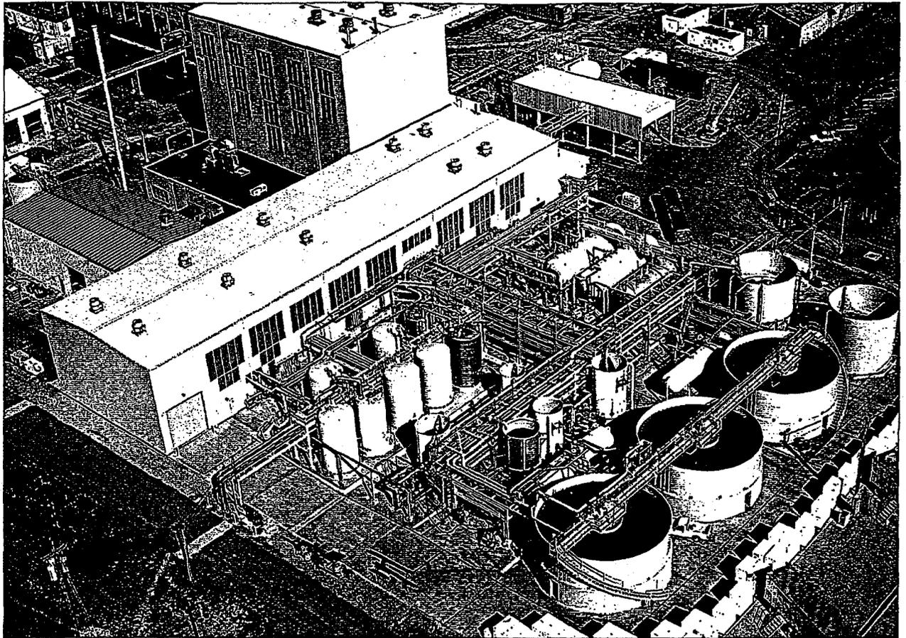
▲ The Advanced Wastewater Treatment facility has a treatment capacity of 2900 gallons per minute. The combined well extraction systems at Fernald pump more than a billion gallons of water from the aquifer each year.
