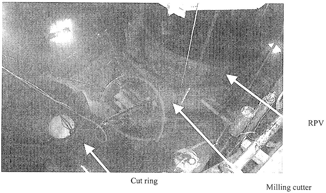
*Figure 5. Dismantling activities during the horizontal cutting.*
