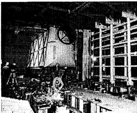
*Figure 3. Dampierre 1 – Condenser module introduction*
