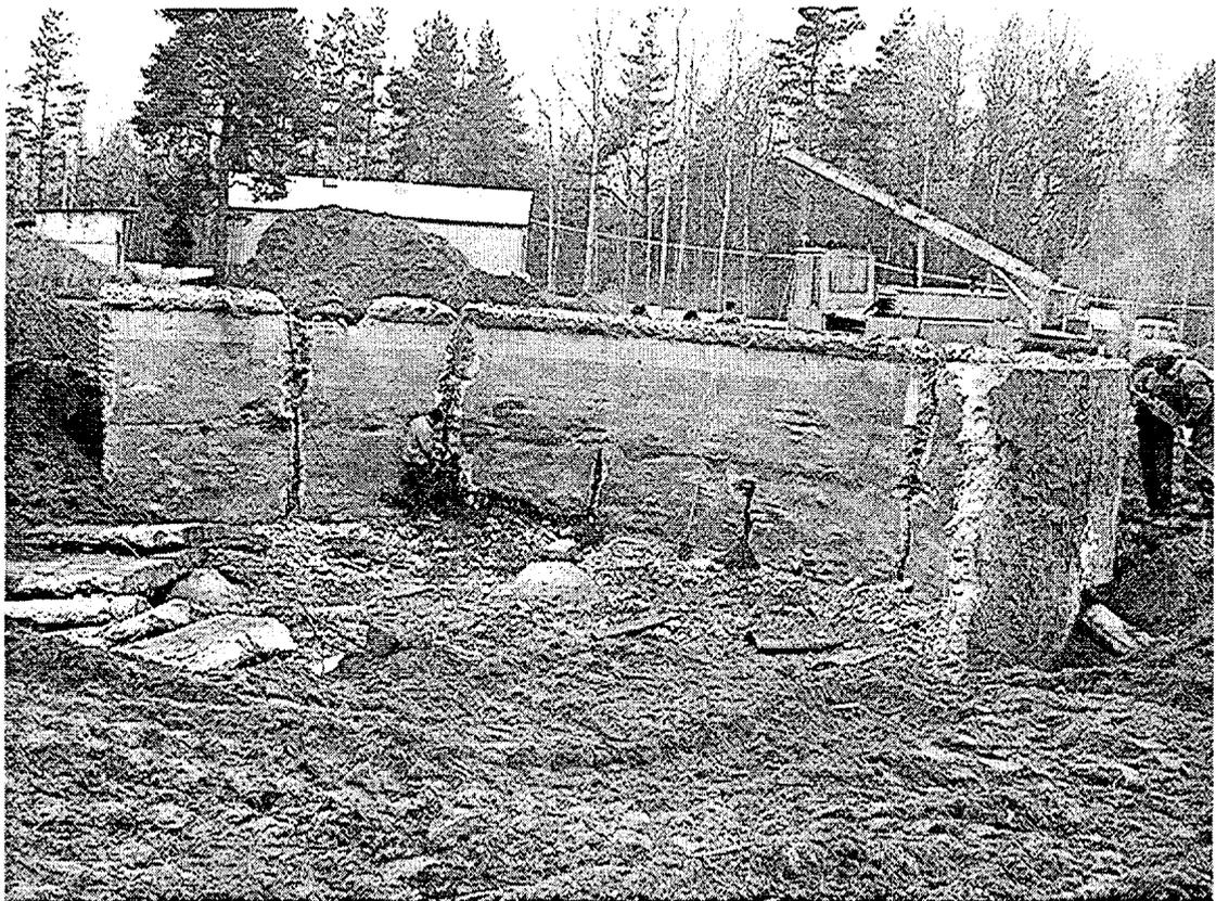
*Fig.4. Dismantling of the unused concrete tank in the SNR yard.*
