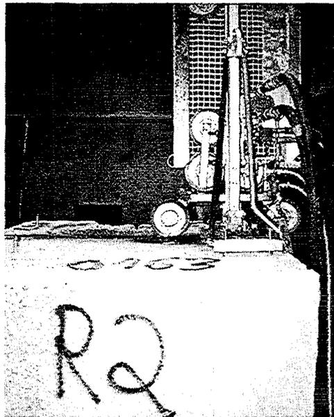
*Fig. 2: Sawing off parts of a concrete bar by a rope saw*
