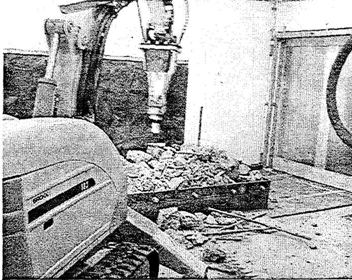
*Fig. 3: Mincing the concrete bars with a power shovel*
