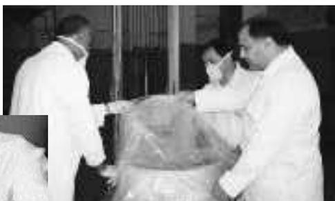
**Cementation of the sludge from chemical treatment.**
