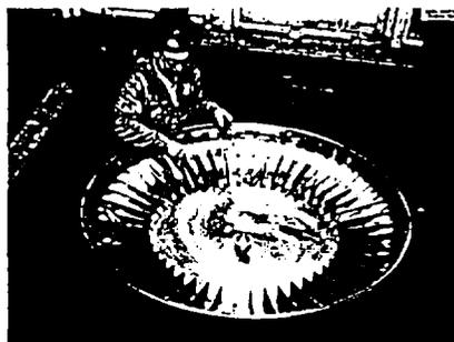
Figure 31. Lower plenum of the MSRE [6]
