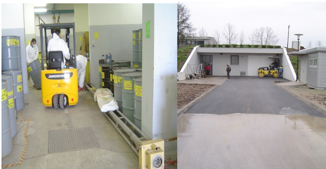
Figure 1 Central Interim Storage for small producers – inside and front side.
