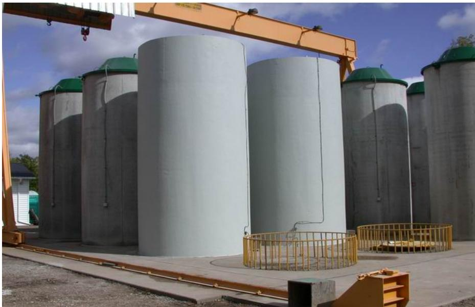
Figure 4: Canisters for storing waste from isotope production.
