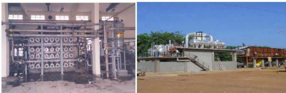
Fig. 1: Hybrid MSF-RO Desalination Demonstration Plant, Kalpakkam
