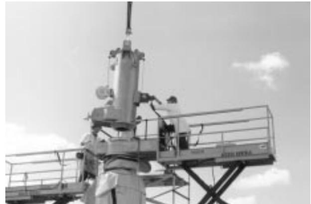
transfer container is returned to the cart and then the spent fuel pool for another loaded basket. A total of six baskets per cask are loaded in this manner.
